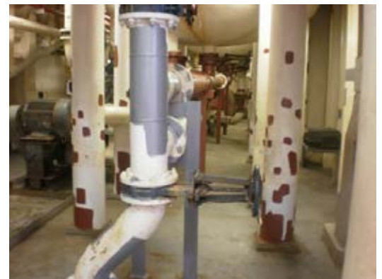
Spot repaired surface on pipeline
