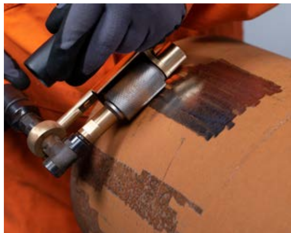
Spot repaired surface on pipeline
