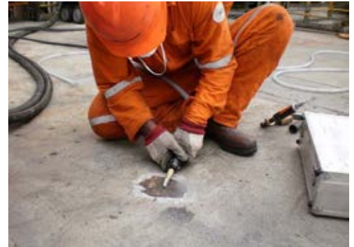
Spot repaired surface on deck
