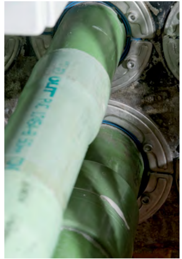
The seals are openable to allow for changes and upgrades.
