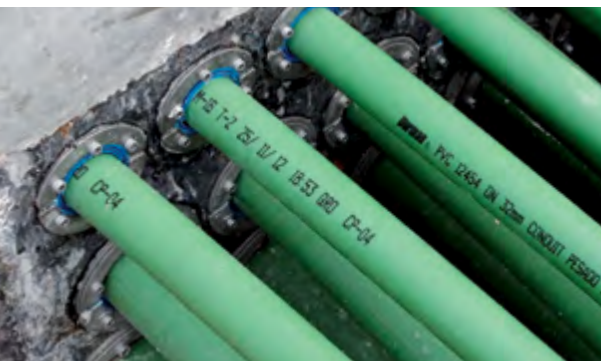
Roxtec seals are adaptable to cables and pipes of different sizes.
