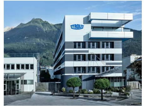
TYROLIT headquarters in Schwaz (Austria)
