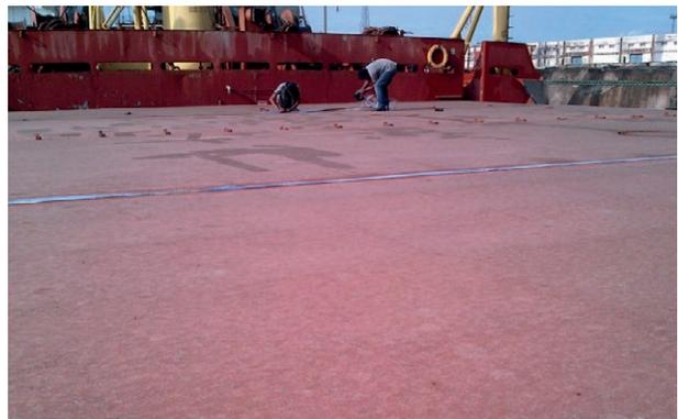
*HatchCover tape being applied on a vessel*
