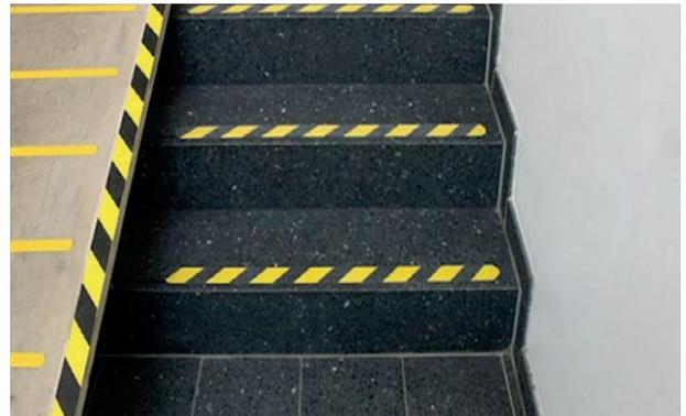
SlipStop tape applied on a staircase
