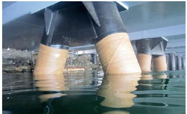
*RustStop applied underneath a bridge*
