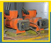
pumps, Stillwater converted to Watson-Marlow Bredel pumps for their flocculent, copper sulfate, and xanthate applications.
