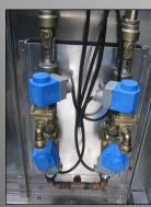
Water is delivered to the adiabatic pre-cooler by the electro-mechanical valve body. The valve assembly is complete with pre adjusted setter devices to assure correct flow rate. The valve body is integrated into the control sequence and pre wired from the factory.
