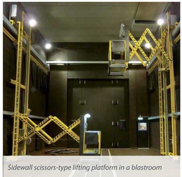
*Sidewall scissors-type lifting platform in a blastroom*
