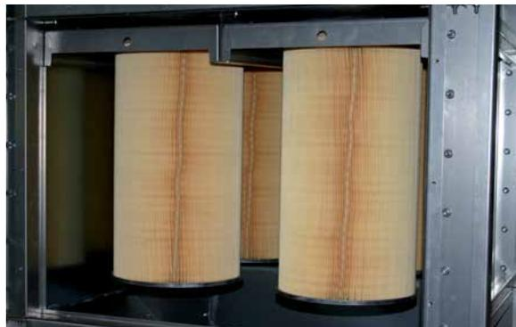
Our cartridge filter unit allows easy replacement of the cartridge filter without entering the raw gas room.
