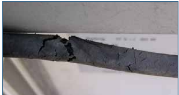
Ozone damage effect
