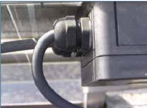
Cable handling misuse - bending radius too small
