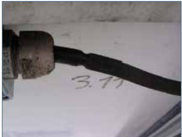
Installation misuse - violent pressure
