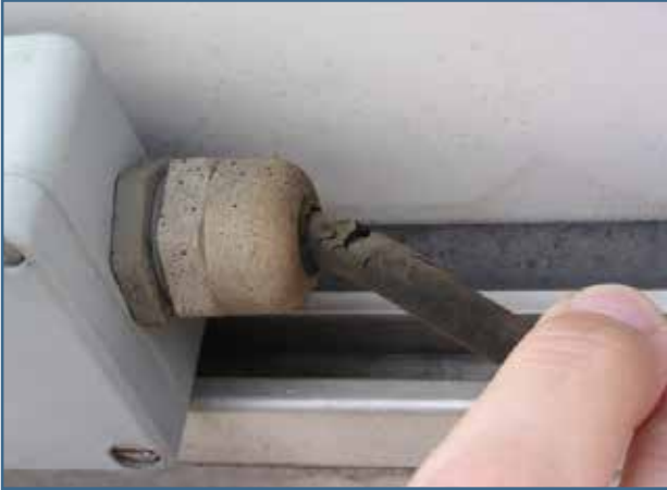
Cable overheating effect
