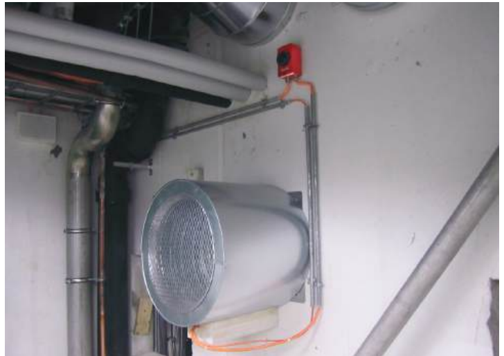
KATKO Firerated switches at Keilaniemi metro station in Espoo, Finland
