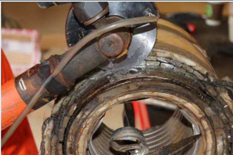
Polyurethane wrapped pipe with carbon fiber enforcement removal
