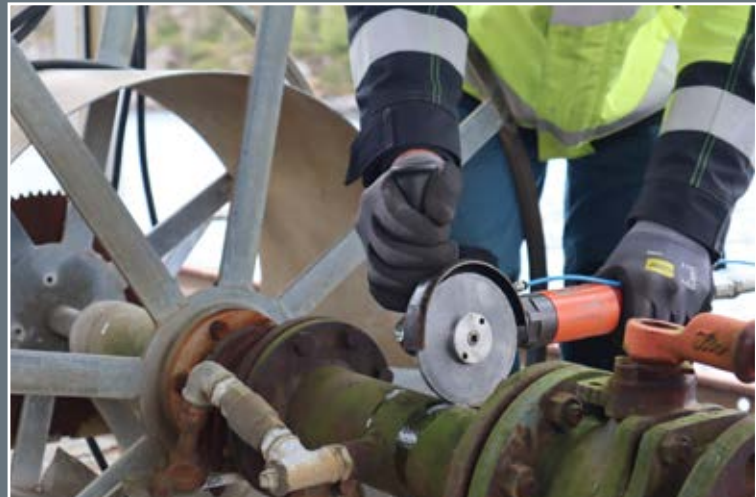
Flange cutting in ATEX Gas zone.
