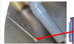
When the sludge is thick, thanks to the slope in our tank, the dry matter accumulates favorably at the low point close to the 200mm diameter rear outlet.
