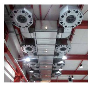
The patented long-range nozzle system developed by us precisely directs heated process air from ceiling level to the operator thus reaching the proper air sinking speeds. This system is especially efficient in connection with the sectional air flow provided by our operator's detection system.
