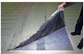
The quick clean system enables a cost-effective and quick cleaning of the paint spraying areas not covered with impact separators. The quick clean foil is drawn to the floor by means of a vacuum in the floor ducts thus adhering here even when walking over it with sticky work boots.
