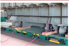
Load is lifted using four synchronized cylinders and set down on transport rollers for further positioning
