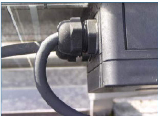
Cable handling misuse - bending radius too small
