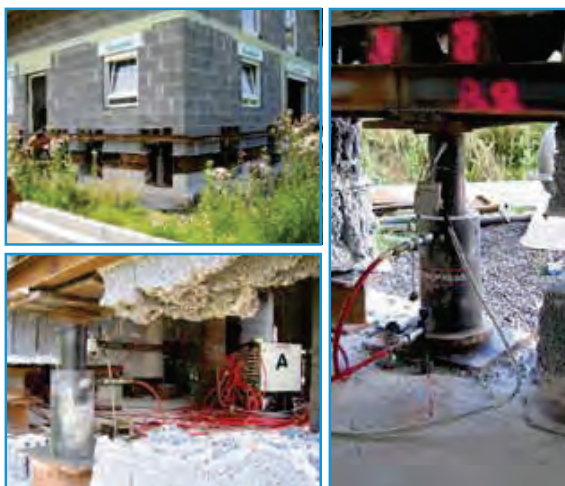
Synchronized lifting with Synchrolift for the rebuilding of house foundations. (Germany 2003)
