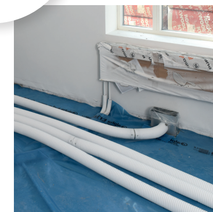
Installation af tilluftsbox under radiator.
