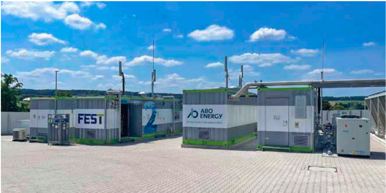
The hydrogen project in Hünfeld-Michelsrombach consists of an electrolyzer, refueling station, and trailer filling station.
