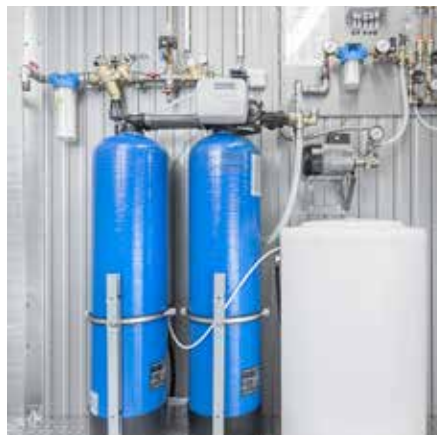
Double softening installation
