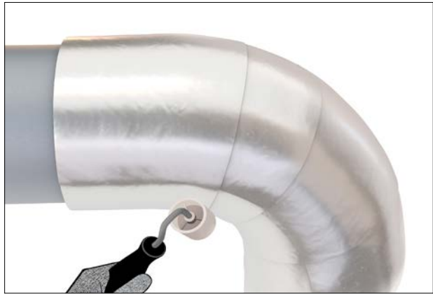
Figure 69: Securing overlaps with roller Using a roller, apply even pressure to all of the overlap seams and joints. Ensure all overlaps are fully secured down without any gaps.
