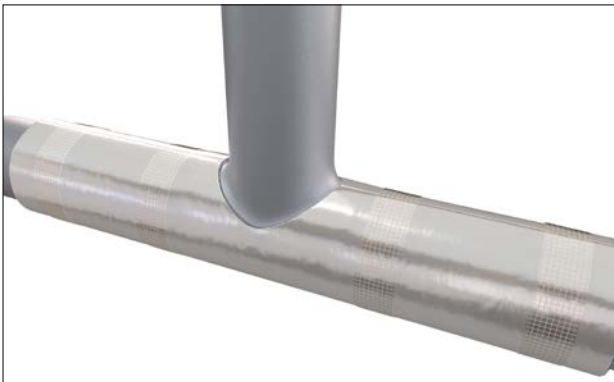
Figure 23: Securing insulation layer with filament tape
