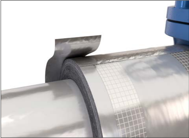
Figure 43: Application of vapour barrier tape at termination Seal the termination ends of the valve body with strips of vapour barrier tape to the outer surfaces of the terminations and the connecting insulated piping surfaces.
