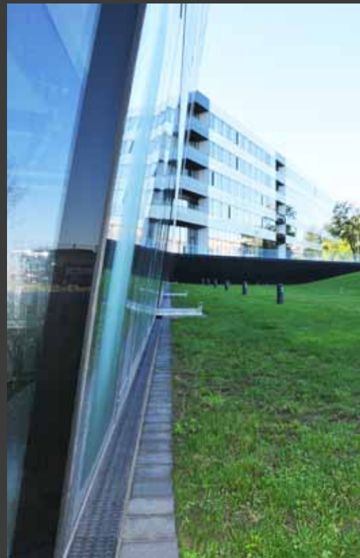
left: The "Laces" connect the individual departments with each other like freely floating bridges bottom: ACO Drain Multiline V 100 G drainage channels with cast iron gratings in the facade area
