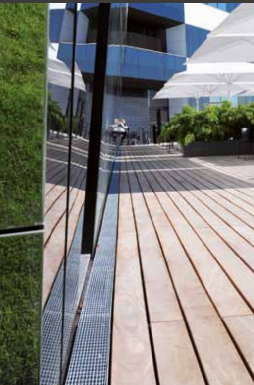
left: Customised structure of ACO drainage channels in front of the facade of the main building
