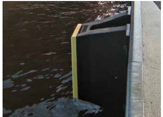
Waterland Terminal | Amsterdam | The Netherlands
