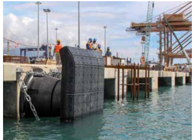
Mauritius Container Terminal | Port Louis | Mauritius
