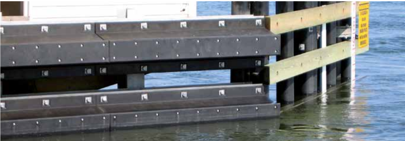
Margate Bridge | Margate City, NJ | USA
