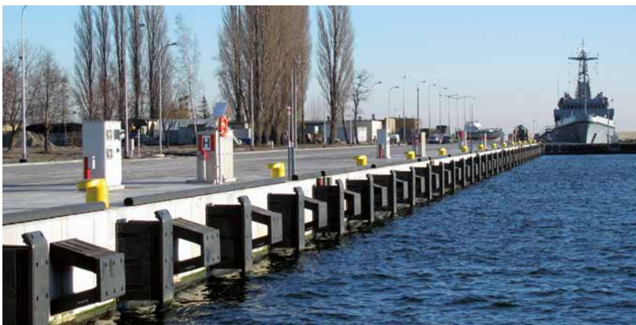
Northern Berth 16 | Port of Gdynia | Poland
