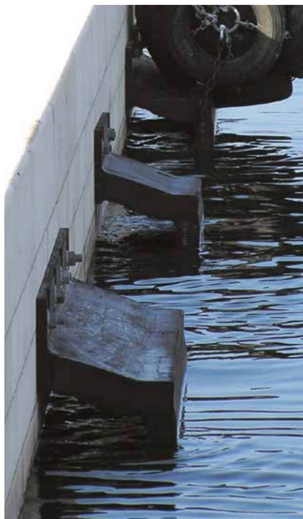
Passenger Terminal | Rijeka | Croatia
