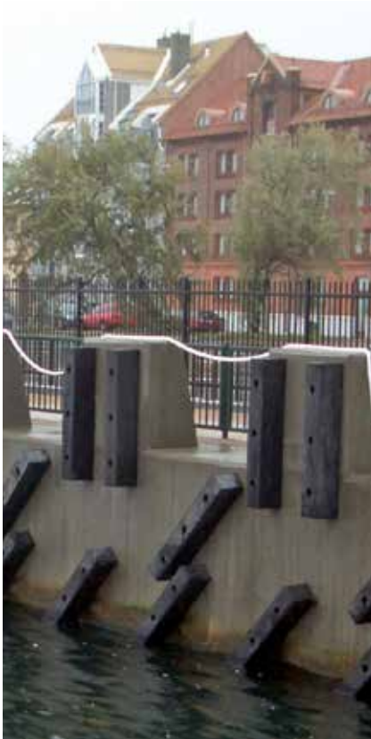
Ferry Terminal | Landskrona | Sweden
