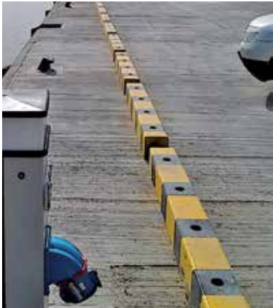
Southern Quay Wall | Simaisma | Qatar
