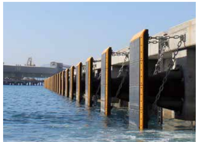
Container Terminal | Aqaba | Jordan
