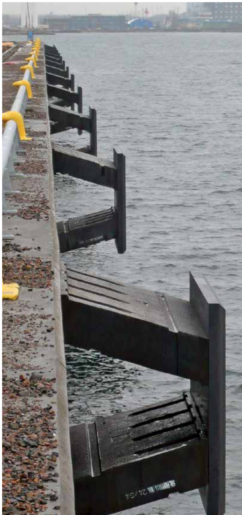
Ferry & RoRo Terminal | Malmö | Sweden
