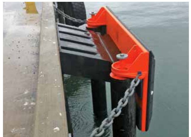
Pier 1 | North Kingstown, RI | USA
