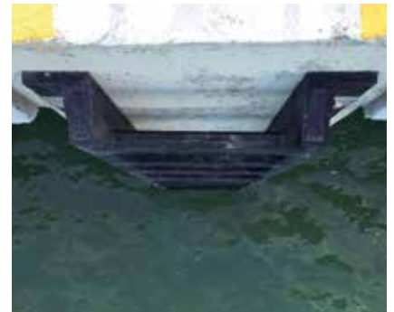
Feed Solid Product Jetty | Johor | Malaysia
