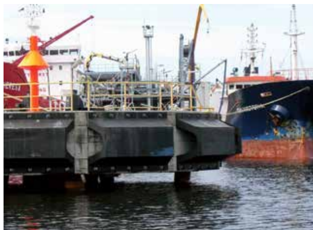
Oil Terminal | Muuga | Estonia
