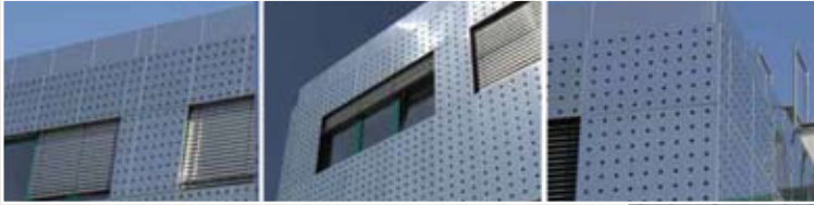
Rustfrie perforerte plater i fasade R40 U120.
