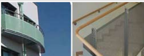
Perforert aluminium, pulverlakkert i mønster R10 T15
