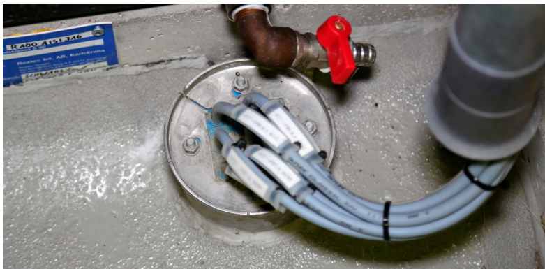
⊕ Roxtec seals protect equipment in the basement from water and humidity.
