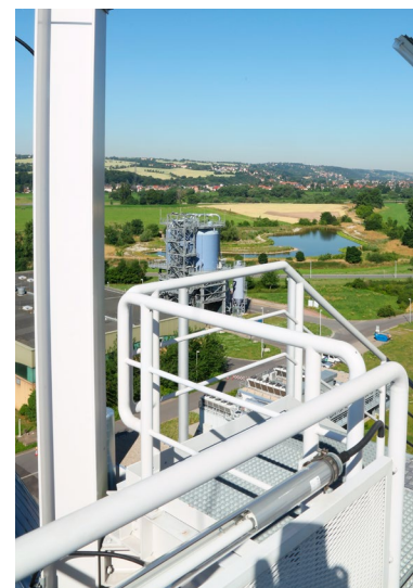
⊕ The Dresden-Kaditz wastewater treatment plant plays an important role for a sustainable development of the society.
