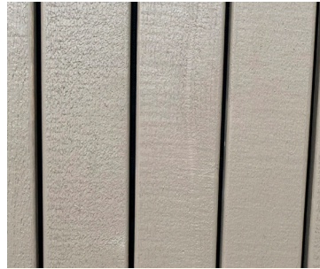
Vertical wood painted siding
