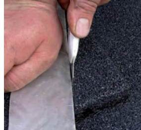
Cut the tiles with a commercially available carpet knife along a steel edge.
