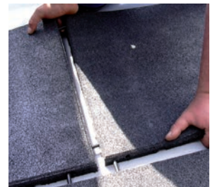
Dowels can be used to fix the tiles to each other.
