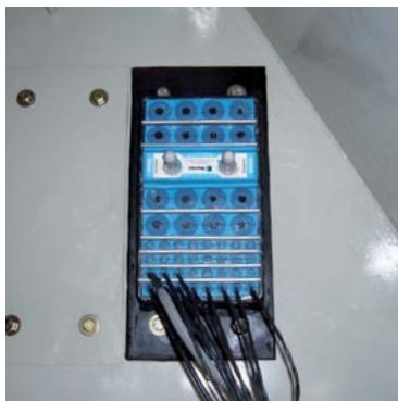
Fire-proof and pressure resistant cable seal.
