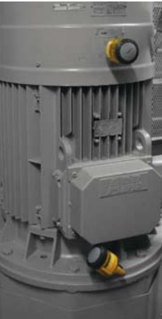
Engine room applications: – fan bearings – electric motor bearings – pump bearings Lubrication system: Klübermatic FLEX 60 cm³ Klübermatic FLEX 125 cm³
