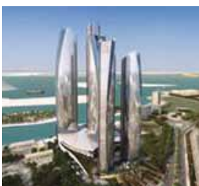
Etihad Towers Abu Dhabi-FAE
