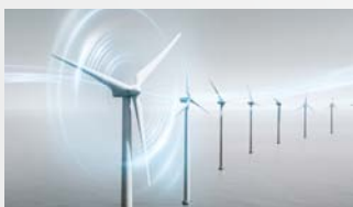
Renewable Energy & Power Generation
