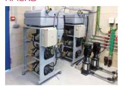
We have water pump racks for a high pressure wash at **70 bar** and **84-126L/min**, with 11 or 16.5kW total power, including respectively- 2 or 3 70bar pumps with 5.5kW power. They include a **200L** water tank at a height to adequately supply the water pumps, and a by-pass valve with a pressure regulator. A 100 micron inlet filter protects the water pumps and prevents nozzles from clogging.
