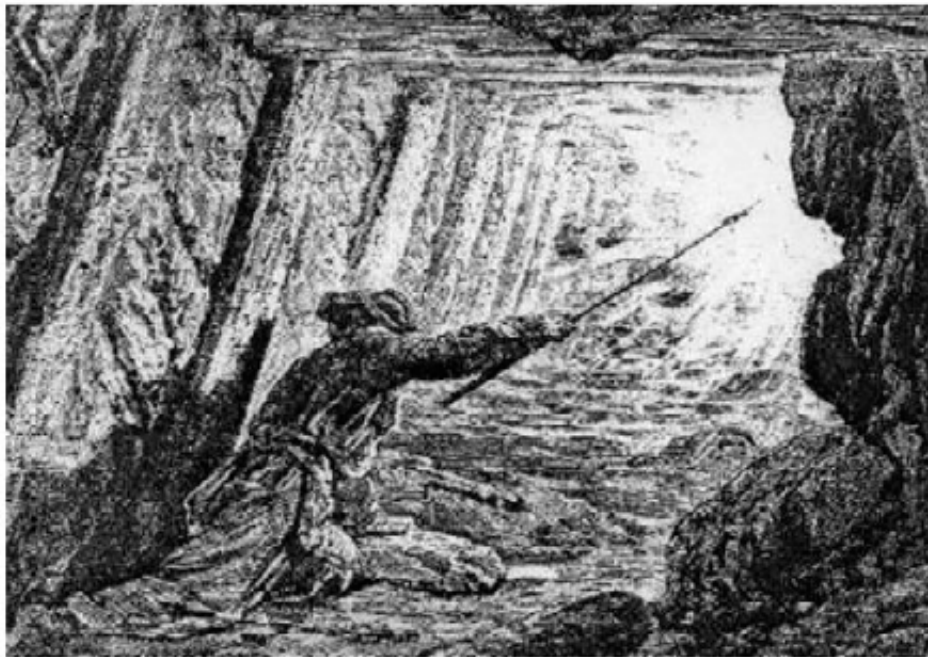
Picture 2: controlled explosions to avoid the accumulation of dangerous gas concentrations inside mines
