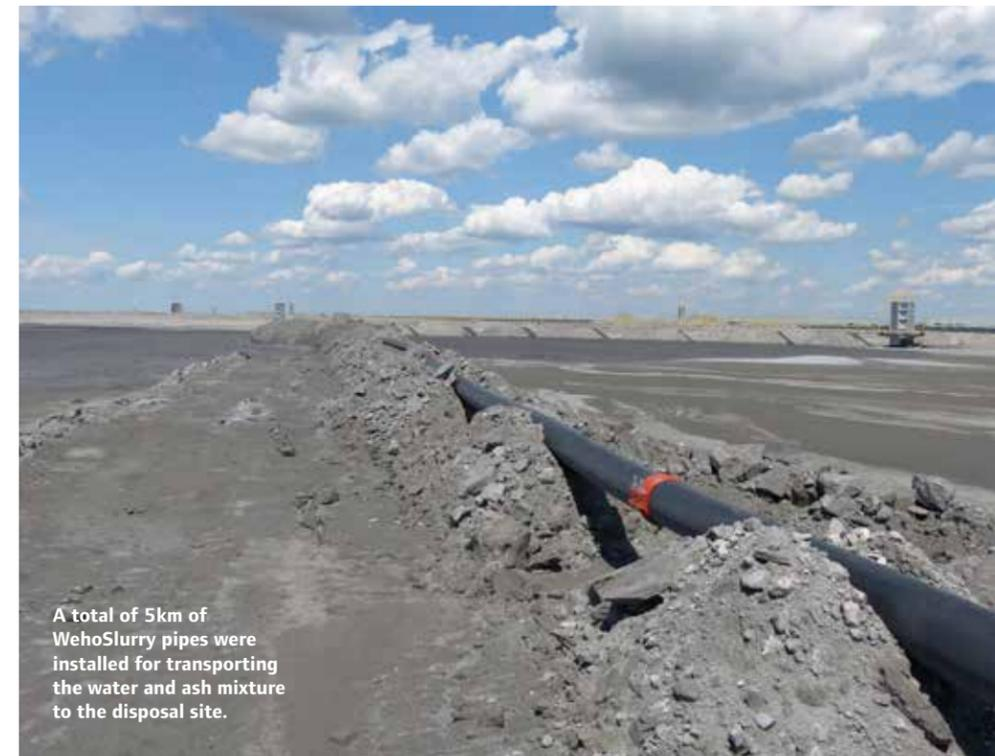
A total of 5km of WehoSlurry pipes were installed for transporting the water and ash mixture to the disposal site.
