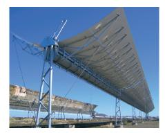
Sections for solar thermal power plants should be able to withstand heavy loads and be easy to maintain.
