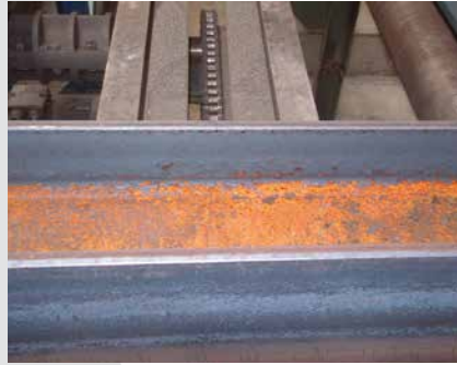
Steel beam before...
