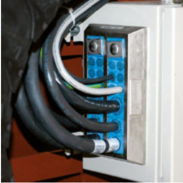
Power supply cabinet: The Roxtec CF 32 can accommodate several cables in a small space.
