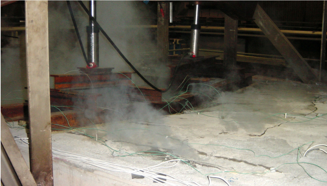
Figure 4. Test H138 in [2]. Cracks in top flange after approx. 15 min. Photo K. Hertz.
