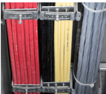
Triax, video and audio cables made by Draka Communications – extreme space ratio and still optimal transmission characteristics.
