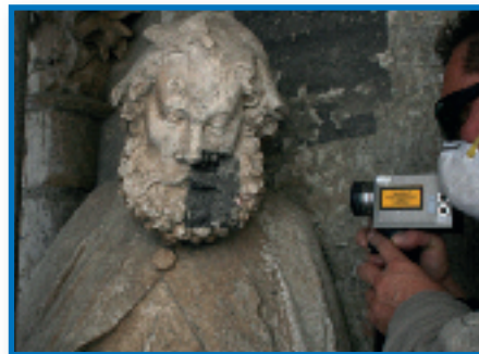
Contaminant & soot removal to restore original finishes
