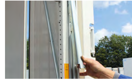
A perforated strip can be used to adjust the roof height in 50 mm steps.
