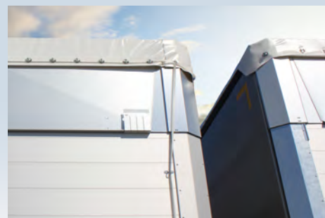
The roof is customs-secure thanks to the bulkhead covering.
