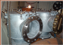
DN 350 bilge water filter Sea-water filters for engine cooling
