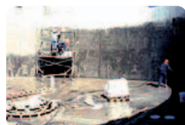
Annacis Island Wastewater Plant repair British Columbia, Canada
