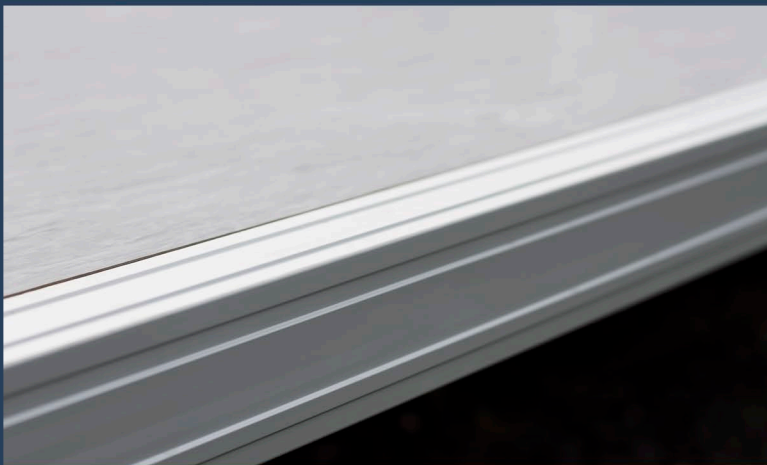
The plywood is sealed off beneath the floor protection.
