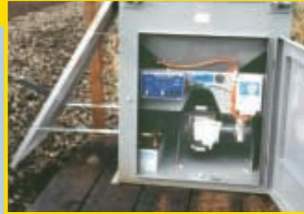
*UK railways experience problems every Autumn when trackside trees shed their leaves. This installation uses a Watson-Marlow Bredel pump to feed gel-borne sand to the rails and increase grip for the trains*
