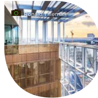
Headquarter Caisse d'Épargne France
