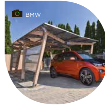
BMW Solar Carport South Africa
