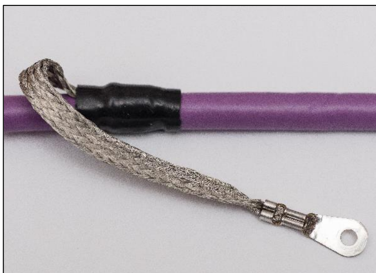
Figure 55: Additional connection of the cable shield (Product Indu Sol, Photo Niemann)
