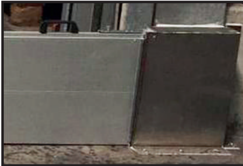
COLUMN RECESSING TO THE COMPARTMENT
