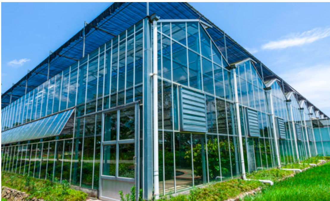
Heating equipment for greenhouses vegetables and flowers
