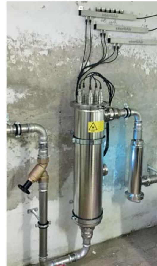
sterilAir® AQD-ST in use for disinfecting spring water, salad washing water and process water.
