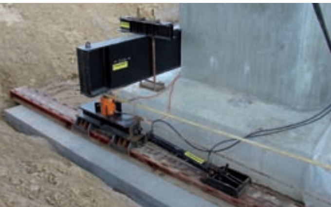
Push system. Skid tracks with oblong holes to accept the shoe for the hydraulic pushing cylinder.
