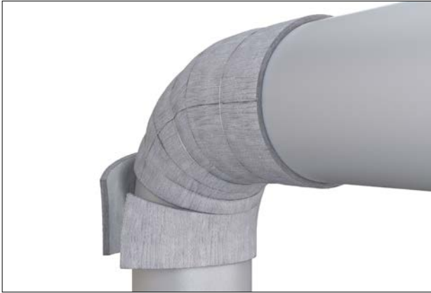
Figure 35: Segment installation.
